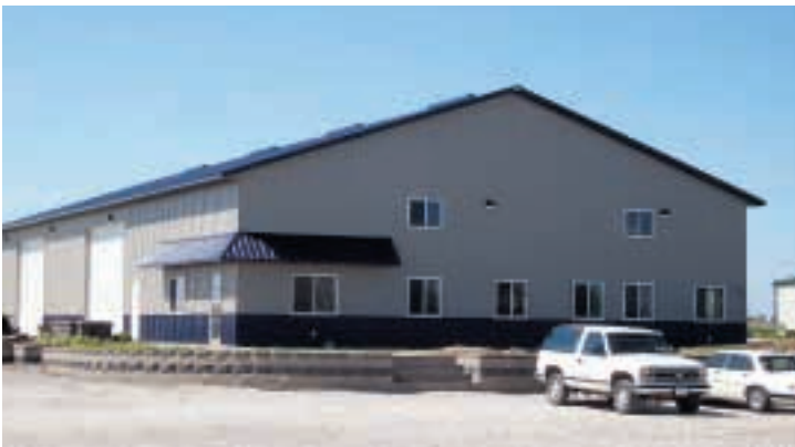
ABC Landscaping, Ames, IA, Rotert Construction, 60' x 120' x 16'
