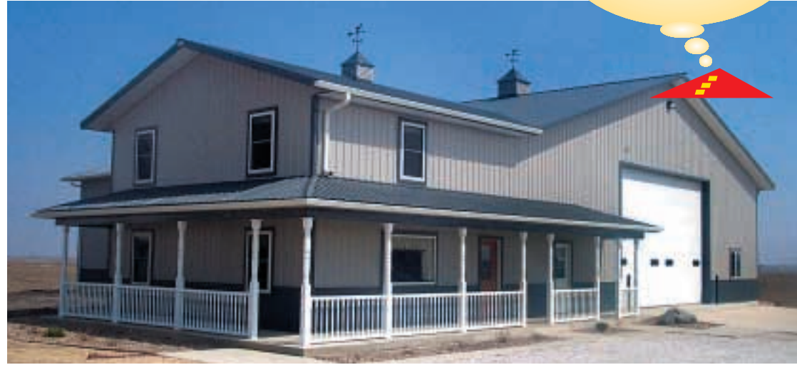
Joe Stevermer, Easton, MN, 60'x180'x16' two-story office/rec room with .060 FRP fully lined shop for power washing.
