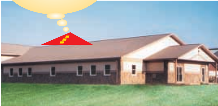
Pearl Creek School, classrooms and gymnasium
