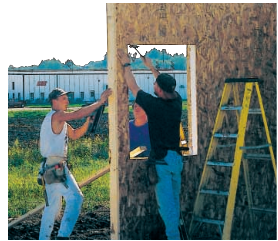
Part of the EPS production facility as seen from a Solid Core Building going up.
